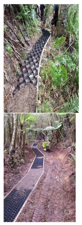
Photos. (Left): 'Presto' Geoweb based system used to stabilise BAM on walking tracks. (Right): 'Jakmat' Geocell system being used to stabilise aggregate walking track surfacing (Photos courtesy of T. Butler, Frame Group Ltd).
